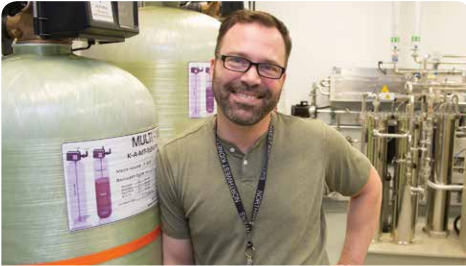
Dan Harris, facilities systems specialist, oversees the new Aquaboss system at our Lake City clinic. The system purifies water for dialysis.
